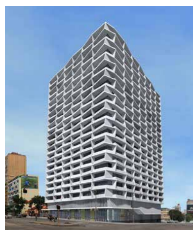
CETA 24 Maputo, MOZAMBIQUE / RESIDENTIAL Arq: PITAGORAS GROUP
